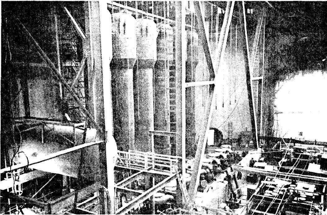
Figure 14 Boilers and Primary Pump Bowls
