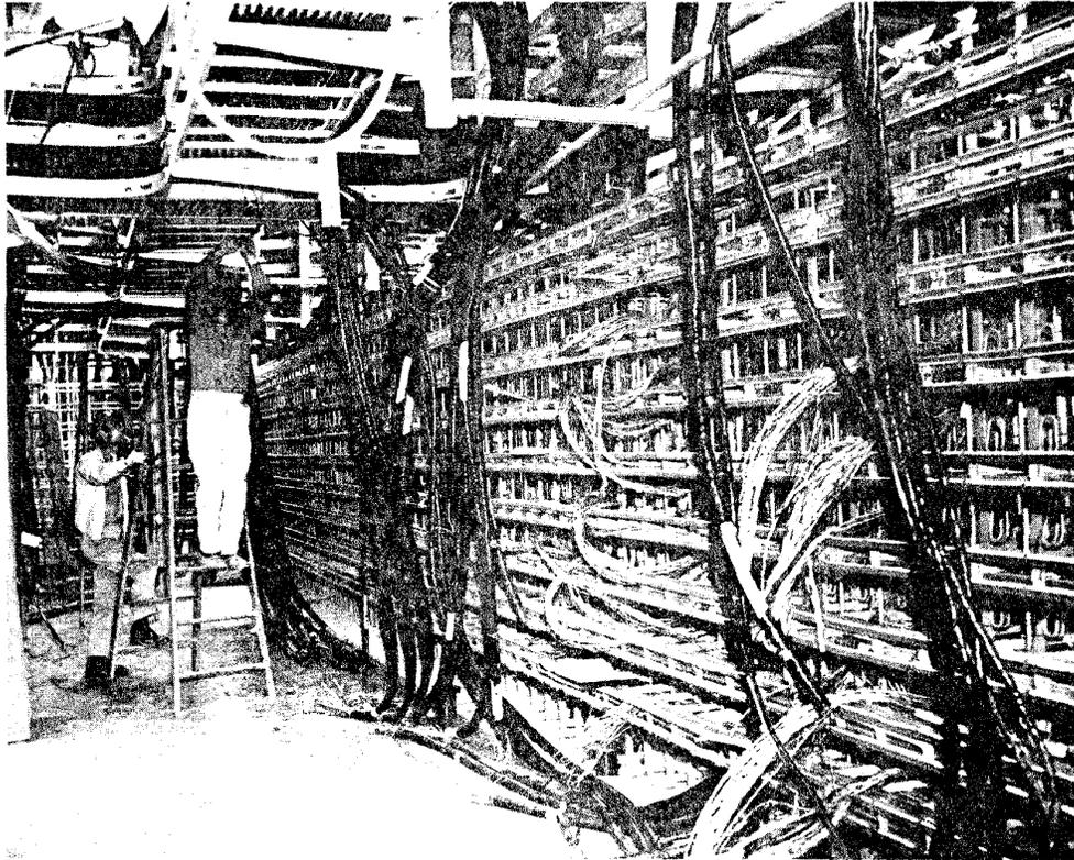
Figure 19 Control Distribution Frames
