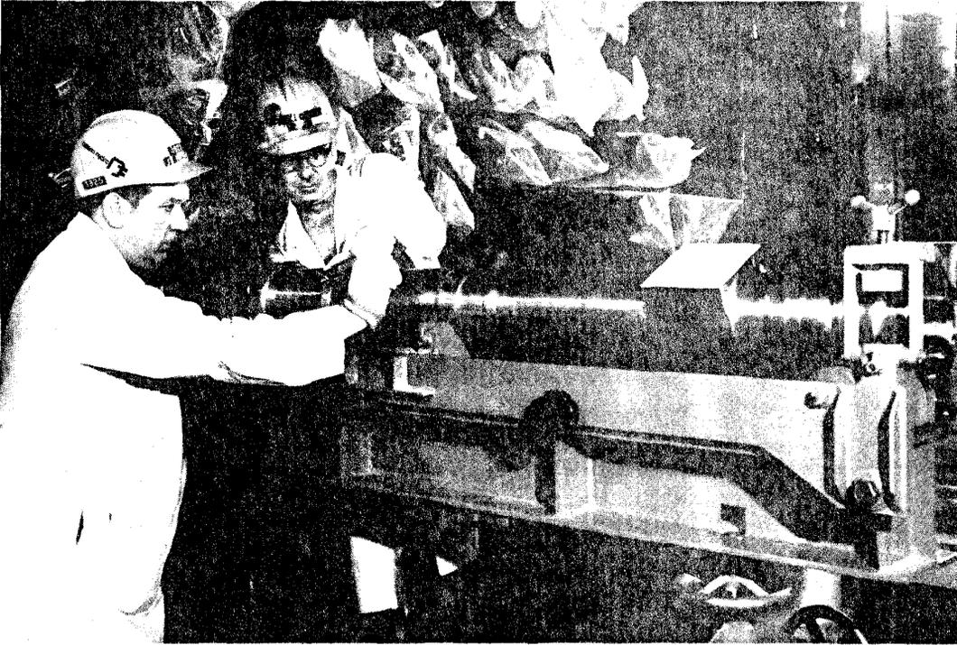
Figure 11 Installing Calandria Tube End Fittings
