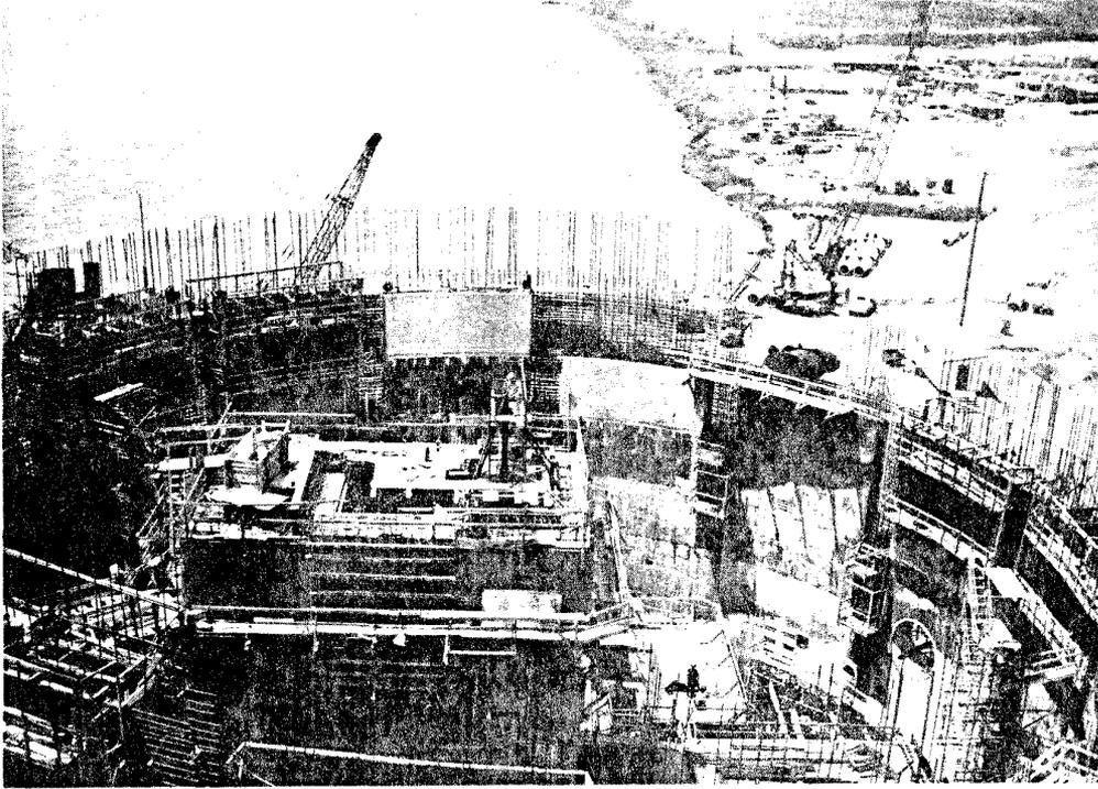
Figure 5 Reactor Building Perimeter Wall Forms
