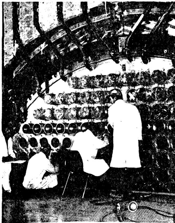
Figure 10 Calandria Tube Sheets Showing Bellows Seal
