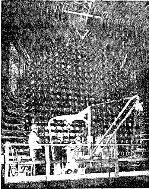
Figure 13 Installing Closure Plugs
