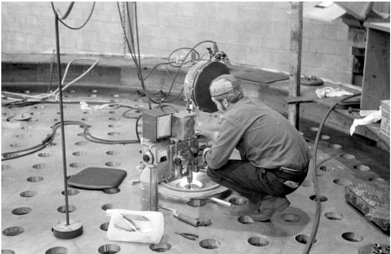
Figure 9 Making the lattice tube to tubesheet weld
