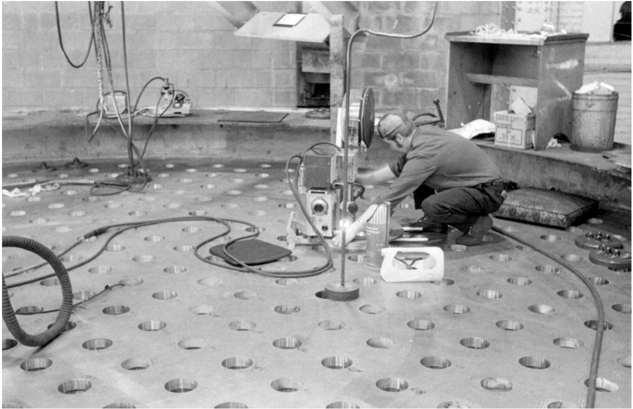
Figure 8 Making the lattice tube to tubesheet weld
