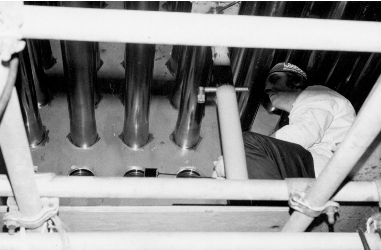
Figure 14 Inside the calandria, during calandria tube i
