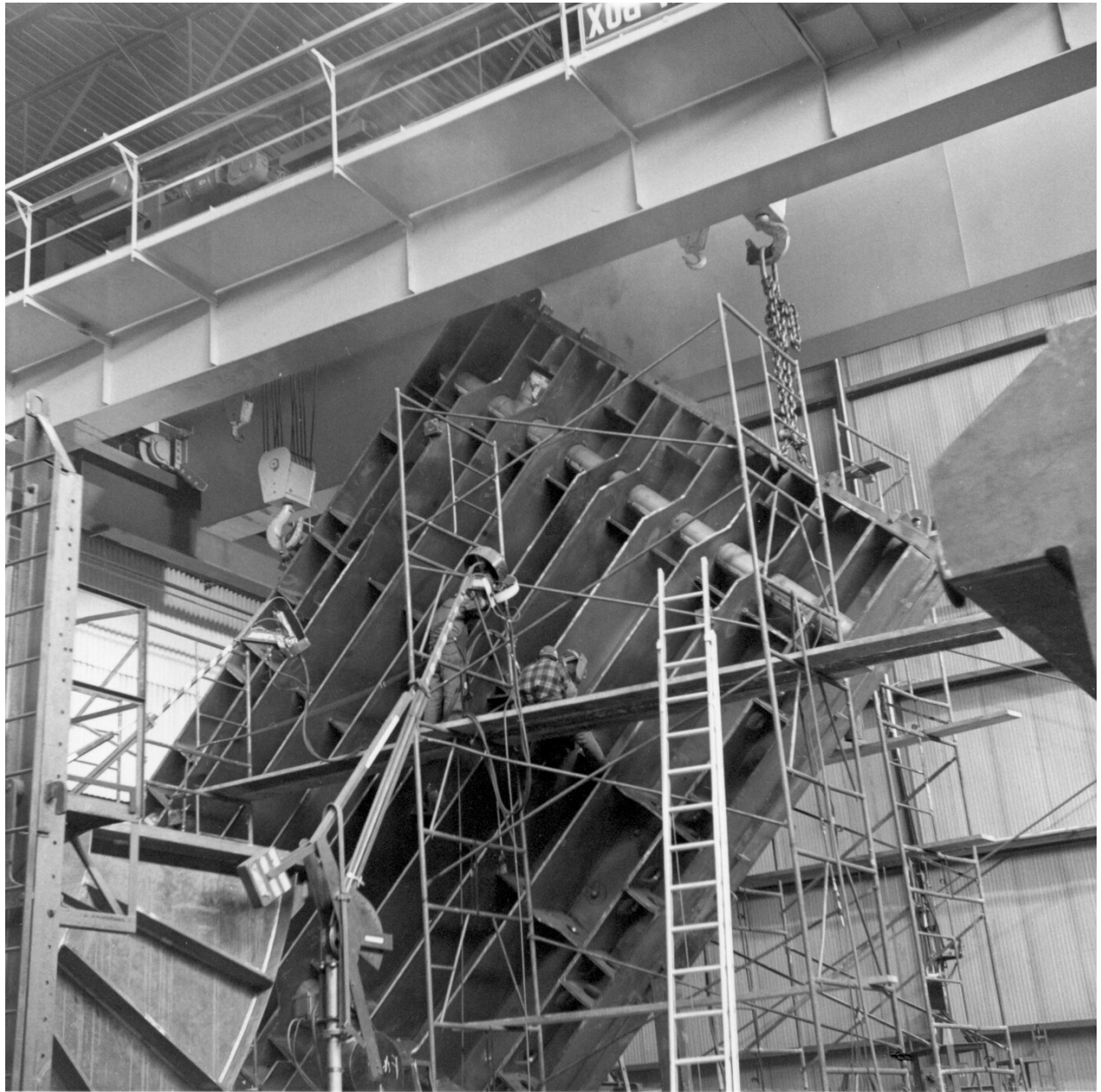
Figure 19 Section of shield tank being assembled.
